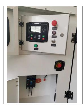
Standard Control Panel is the basic configuration for normal operation and usage. It is of some advantage such as easy to operate various function and well protection. Operative buttons such as Turn On, Per-heart. Starting, Stop (Emergency Stop) on the panel. while malfunction occurs, control panel will stop the generator and also alarm with light or buzz.
