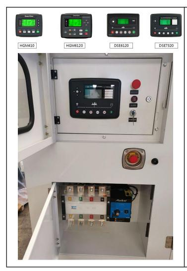
Automatic Control Panel is the basic configuration for nobody on duty controlling generator. This kind of panel can accept the remote Start/Stop signals.
