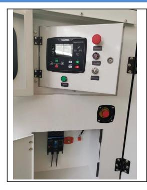
Standard Control Panel is the basic configuration for normal operation and usage. It is of some advantage such as easy to operate various function and well protection. Operative buttons such as Turn On, Per-heart. Starting, Stop (Emergency Stop) on the panel. while malfunction occurs, control panel will stop the generator and also alarm with light or buzz.
