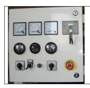
Standard Control Panel is the basic configuration for normal operation and usage. It is of some advantage such as easy to operate various function and well protection. Operative buttons such as Turn On, Per-heart. Starting, Stop (Emergency Stop) on the panel while malfunction occurs, control panel will stop the generator and also alarm with light or buzz.
